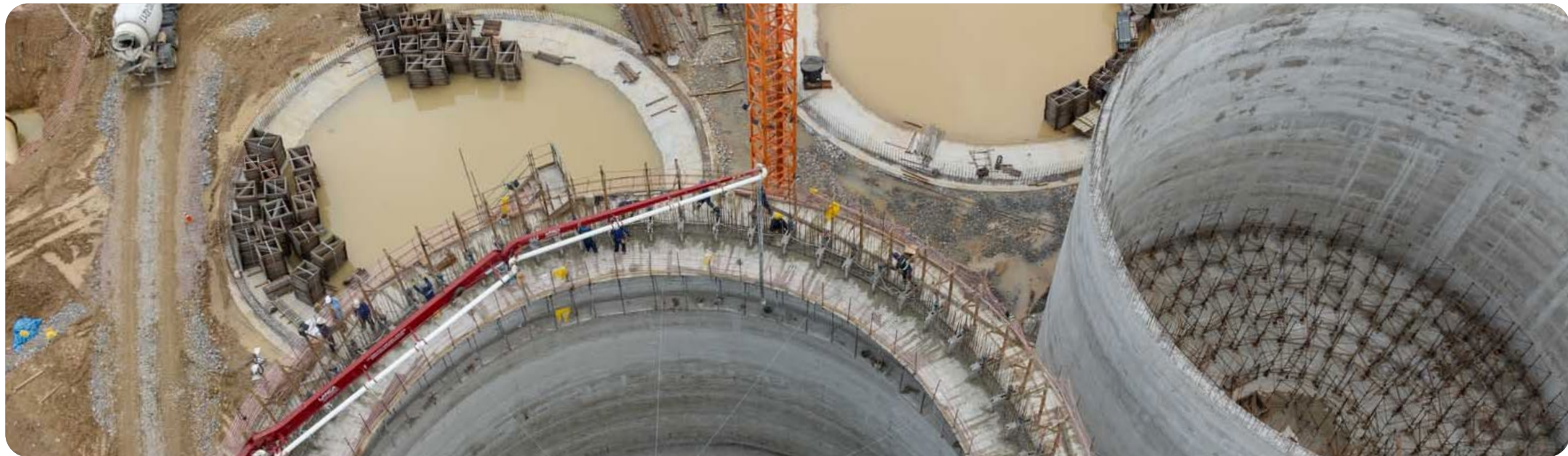
Atuba Sul STP works - Photographer: André Thiago Chaves Aguiar
