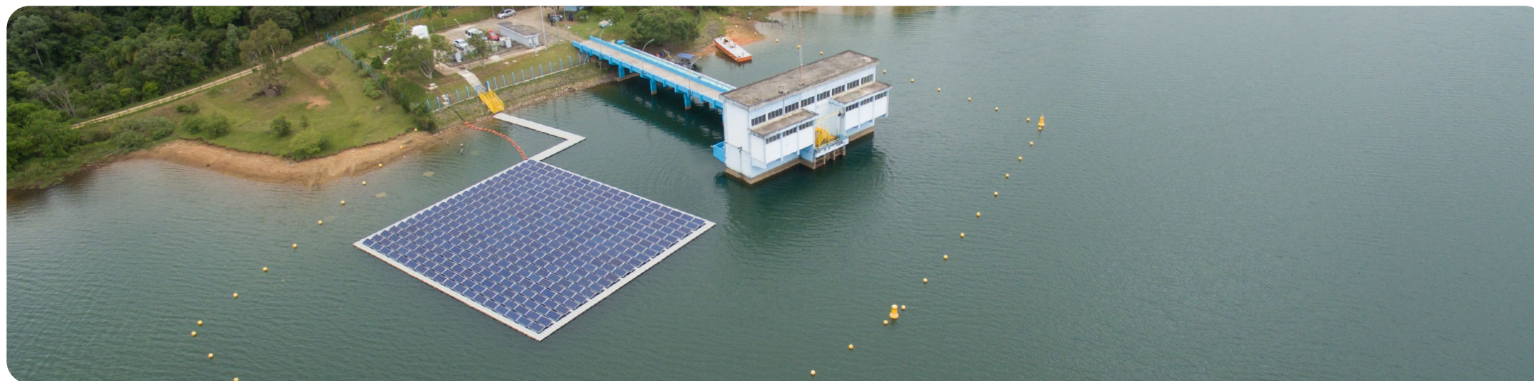
Passauna WTP by drone - Photographer: André Thiago Chaves Aguiar
