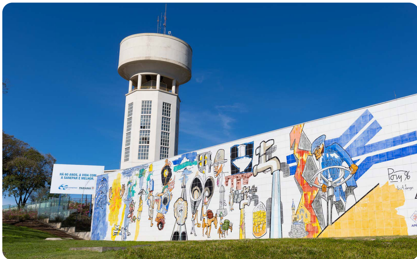
Alto da XV Reservoir - Poty Lazzarotto Panel - Photographer: André Thiago Chaves Aguiar
